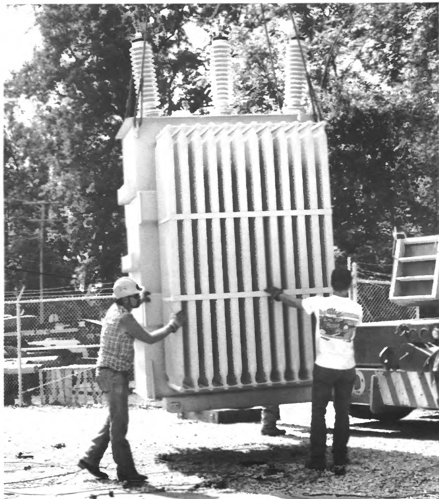
Norris employees stabilize a transformer as it's hoisted into place.
