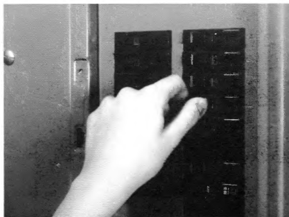
Breakers such as these are more convenient than fuses: if they trip often, you still have problems.
