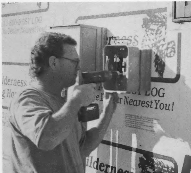
Dave Behrens, an employee of Smith Electric, installs a meter base.
