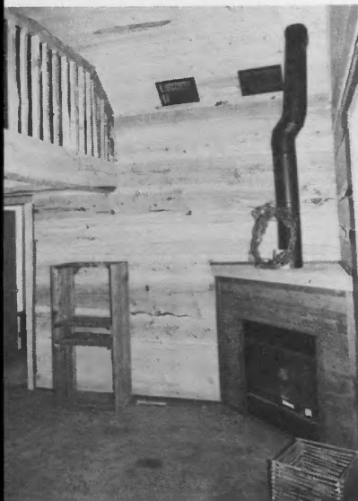
An interior view of one of the cabins, showing the fireplace. These cabins are all hand-made, with dove-tail cuts; they are not kits.
