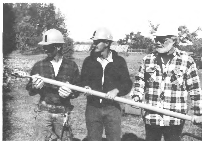
Construction foreman/instructor Dick Albert (right) explains to linemen apprentices Steve Rosenthal (left) and Mike Butler the business end of a "hot stick" used to work on and with high-voltage lines.
