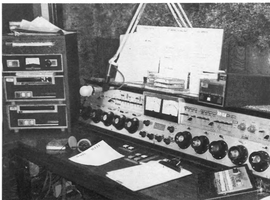
Main control room displays sophisticated electronic equipment.
