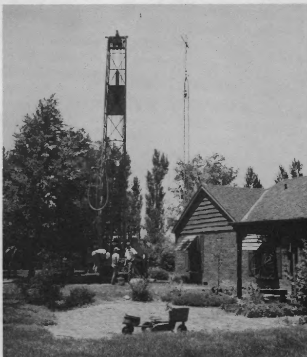
Employees of Snell Heating and Air Conditioning installing one of four 150-foot wells for the Satoriuses' geothermal heating and cooling system.
