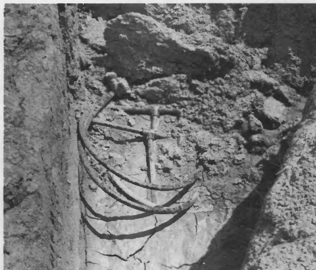
Exposed section of piping
