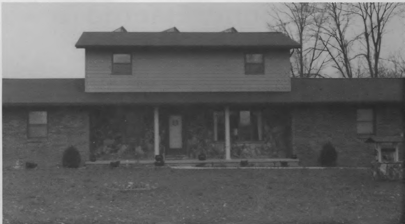
The Littekens' all-electric home is situated just west of Aviston, right off old Rt. 50. The wooded area off to the right (south of the home) provides lots of shade and cool breezes, giving them the luxury of low electric bills last summer.
