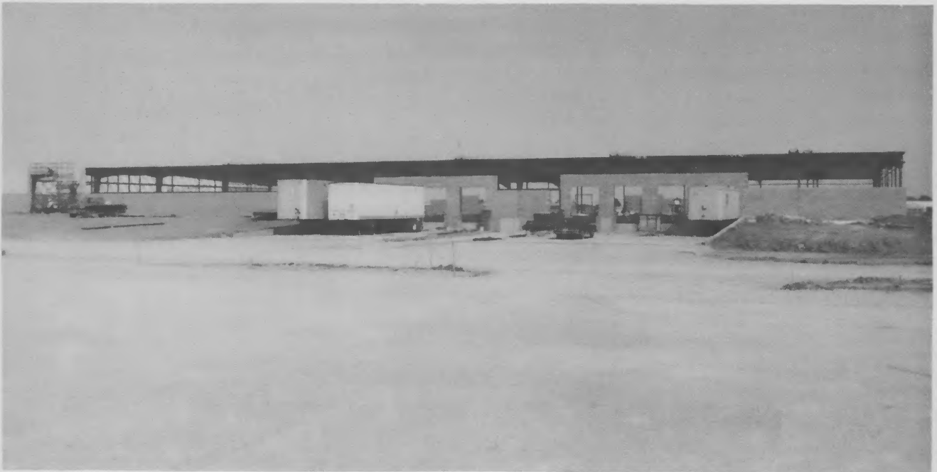
B&M Manufacturing Co.'s plant under construction
