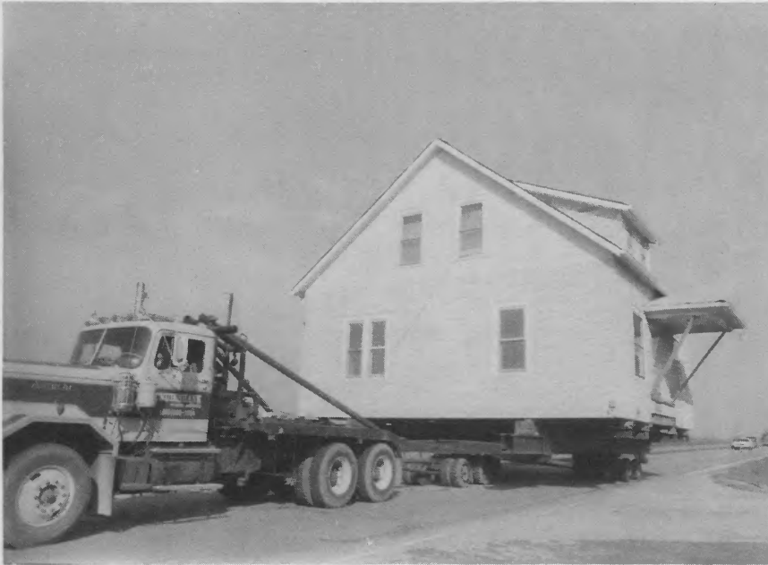
Moving at a snail's pace to avoid structural damage to the house, Cruikshank House Moving Co. of East St. Louis travelled south on Rt. 160 to get to the final destination—Kloos Subdivision.
