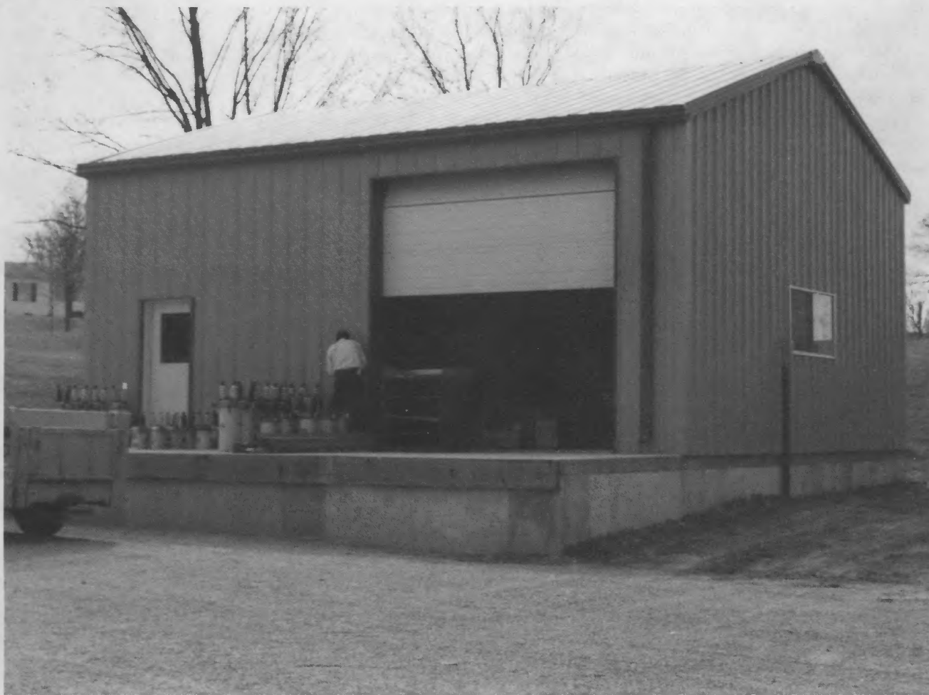
The new reclosure building behind cooperative headquarters is being readied for use.
