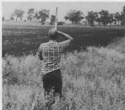
Pilcher, at left with surveyor's rod, and Peterson, at transit, do preliminary work for a line replacement job.
