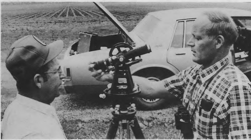
Evan Peterson (left), assistant engineer, substations, and Larry Pilcher, assistant engineer, staking, adjust the surveyor's transit.
