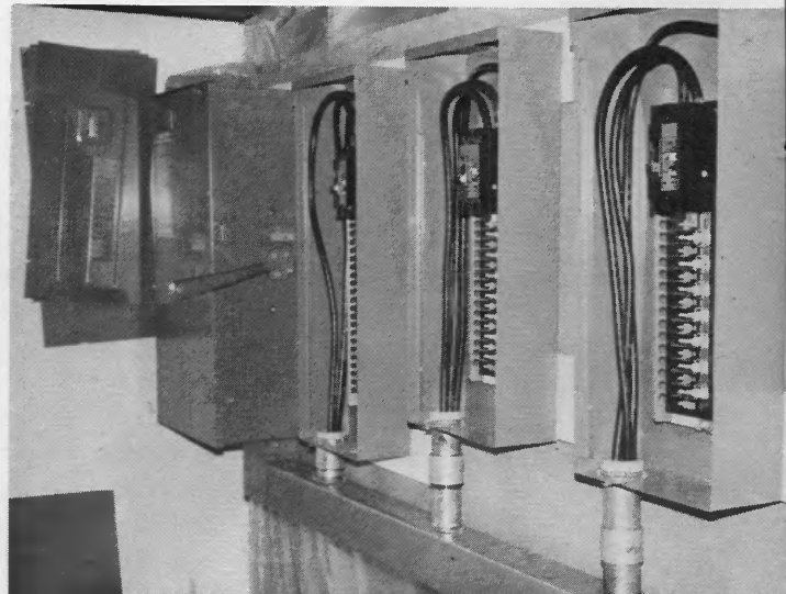
When standard metal service equipment is used, locate it in a clean dry room adjacent to livestock rearing area. Conduit should enter side or bottom with ends sealed.
