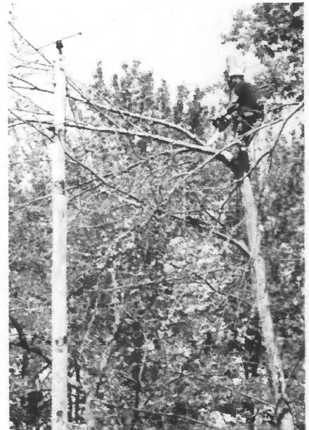
Finishing off the top
