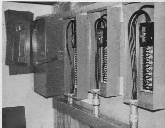
When standard metal service equipment is used, locate it in a dry room adjacent to livestock rearing area. Conduit should be on side or bottom with ends sealed.
