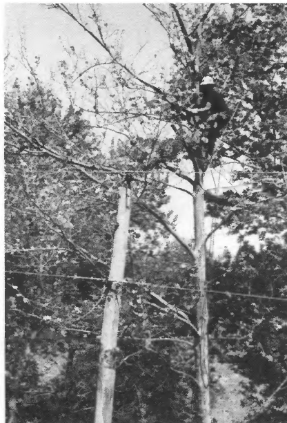
In position to start trimming
