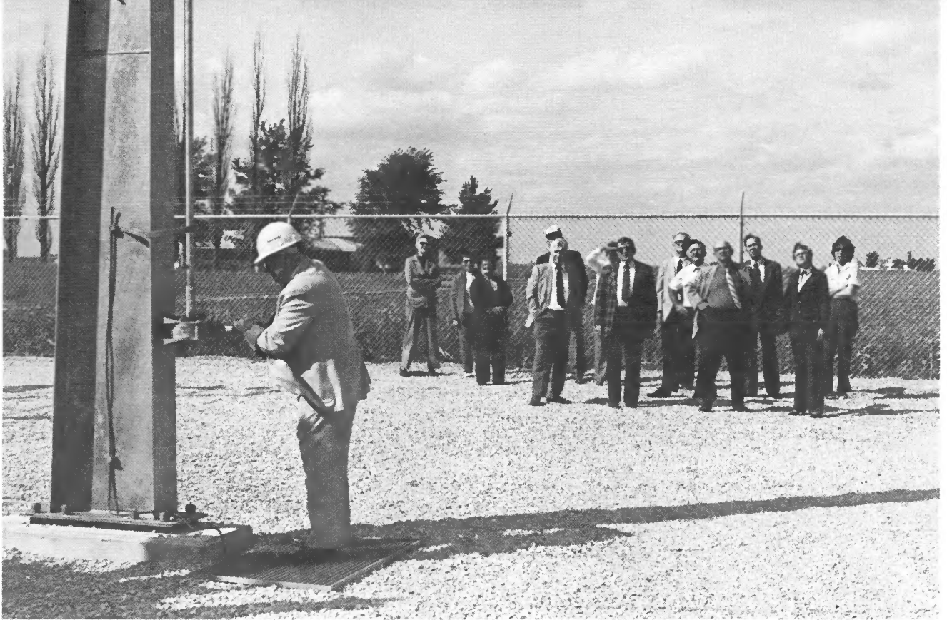
A two-year building project was completed in September when Walter R. Smith, foreground, and members of the board of directors switched into service two new substations in the Garrett and Longview areas.
