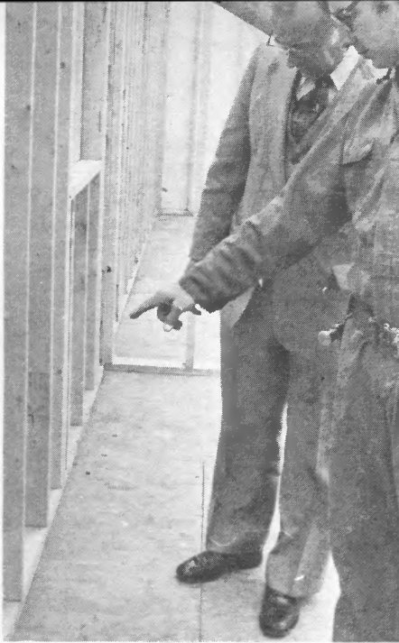
Above, building trades instructor Steve Durian points out the double wall construction of the new house to Edgar Arnn, manager of FMEC. At right, he demonstrates the quilted window covers that help retain heat after the sun sets.
