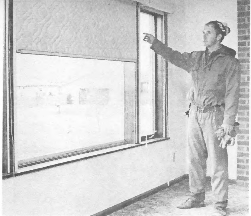
Above, building trades instructor Steve Durian points out the double wall construction of the new house to Edgar Arnn, manager of FMEC. At right, he demonstrates the quilted window covers that help retain heat after the sun sets.
