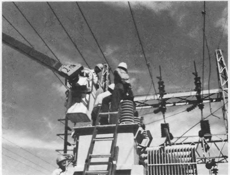
Crews install 5,000-KVA transformer to handle increased load.
