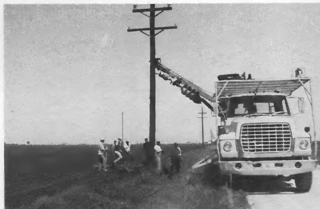
Transmission line pole is set into place.
