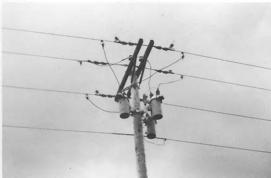
The three-phase breaker installation protects the system from the breakers to the substation. When a fault occurs beyond the breaker it will isolate the line from the source. When the fault is cleared the breaker can be closed and service restored. All 515 breakers on Corn Belt's system have been recently tested and the coordination verified. This should improve your service and is part of our on-going preventative maintenance program.
