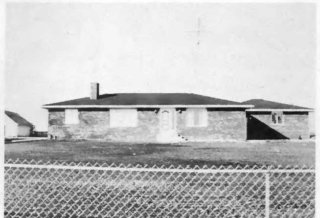
Gilbert Coffey Edinburg, IL Electric Furnace
