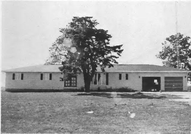
Preston Bennett R.R. 1, Windsor, IL Ceiling Cable
