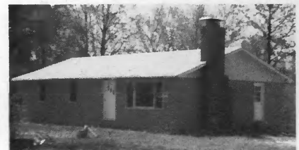
Mr. and Mrs. Paul Ross 3 1/4 Miles Northeast of Lively Grove Built in 1975 1293 Square Feet of Living Area Electrical Contractor—Homeowner
