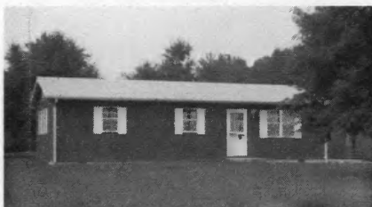
Mr. and Mrs. Forrest Martin 1 Mile Southwest of Salem Built in 1972 1056 Square Feet of Living Area Electrical Contractor — Wayne Bundy
