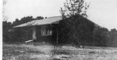
Mr. and Mrs. William Peacock 2 Miles Northeast of Mt. Vernon Built in 1975 2020 Square Feet of Living Area Heating Contractor—Lyle Woods
