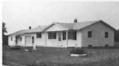
Mr. and Mrs. Dominic Bauza 1½ Miles North of Oakdale Built in 1974 1076 Square Feet of Living Area Electrical Contractor — Dominic Bauza, Jr.
