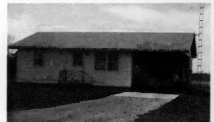
Mrs. Marie Ritter 6 Miles Southeast of Alma Built in 1975 825 Square Feet of Living Area Electrical Contractor—Ray Griffin
