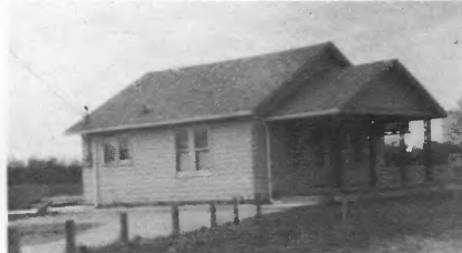
Mr. and Mrs. Russell E. Cooper, Sr. 4½ Miles East of Salem Converted to Electric Heat in 1974 588 Square Feet of Living Area Electrical Contractor—Ted Cantrell
