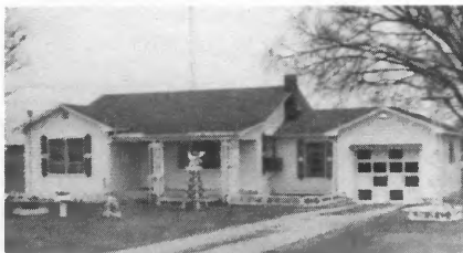
Mr. and Mrs. Harry Phelps ¼ Mile North of Iuka Converted to Electric Heat in 1967 1071 Square Feet of Living Area Electrical Contractor—John Ellis
