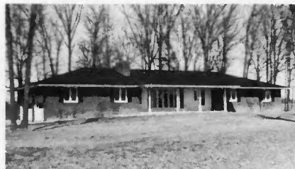
Mr. and Mrs. Kenneth Neilson 1 Mile East of Alma Built in 1974 1610 Square Feet of Living Area Electrical Contractor—Homeowner
