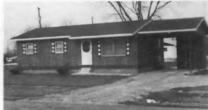
Mr. and Mrs. Edward Glen Dalby Opdyke Built in 1974 883 Square Feet of Living Area Electrical Contractor—Bob Wheeler
