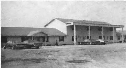
Purcell's Apartments 1 Mile South of Salem Built in 1974 8 Units Electrical Contractor—Purcell Devel. Co.
