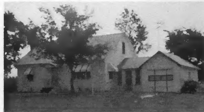
Mr. and Mrs. Leonard Billmeier 1½ Miles South of Caspars Converted and Added to Electric Heat — 1973 2008 Square Feet of Living Area Electrical Contractor — Paul Warner
