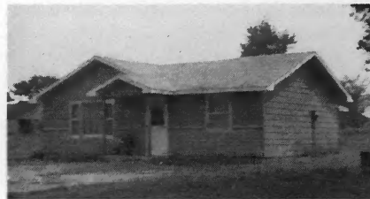
Mr. and Mrs. Loren Bumpus 2½ Miles North of Spring Garden Converted to Electric Heat in 1974 2771 Square Feet of Living Area Electrical Contractor — Lawrence Hall
