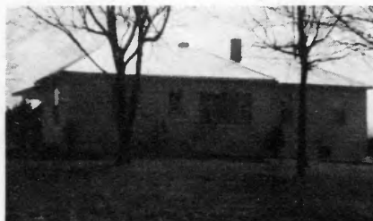
Mr. and Mrs. Beachy Sawyer 4 Miles Northeast of Kell Converted to Electric Heat in 1975 859 Square Feet of Living Area Electrical Contractor—Harvey Mays
