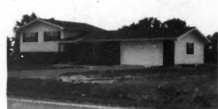
Mr. and Mrs. Paul Pennington 3½ Miles East of Waltonville 1575 Square Feet of Living Area Built in 1975 Electrical Contractor Bill Beasley
