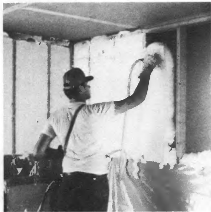
Applying Rapco Foam insulation in wall space of new home.
