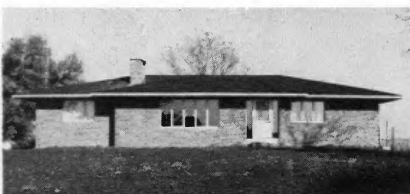
Mr. and Mrs. Charles Jones Edinburg, Ill. Ceiling Cable
