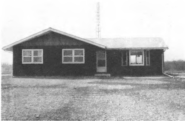
Edward Zulauf Taylorville, Illinois Electric Furnace
