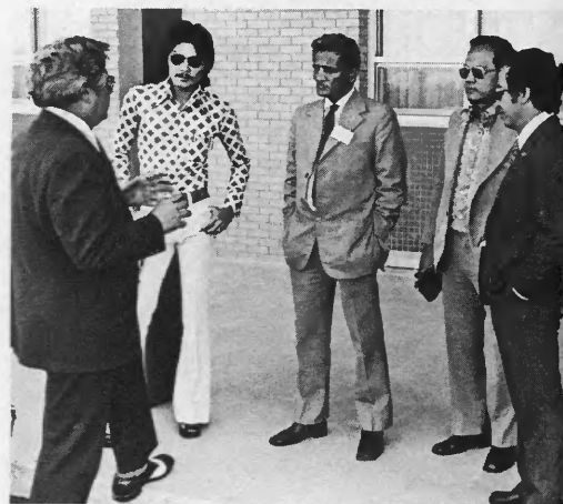
TOP: The trainees gave a cooperative line crew a hand with a sticky conduit coupling. ABOVE: Manager LeRoy Hard discusses the day with visitors, prior to an outing in St. Louis. RIGHT: The group watches a line crew finish wiring the transformer installation.
