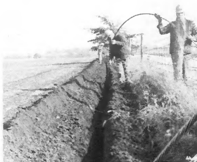
Darrell Boston operates the trenching machine to prepare for the laying of three-phase underground cable and members of the line department install the cable in the trench.
