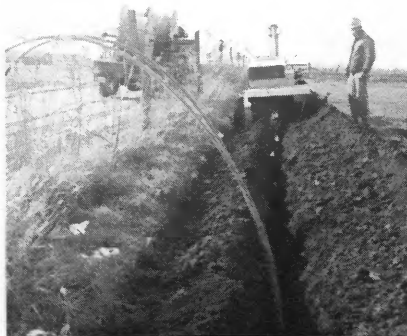
Darrell Boston operates the trenching machine to prepare for the laying of three-phase underground cable and members of the line department install the cable in the trench.
