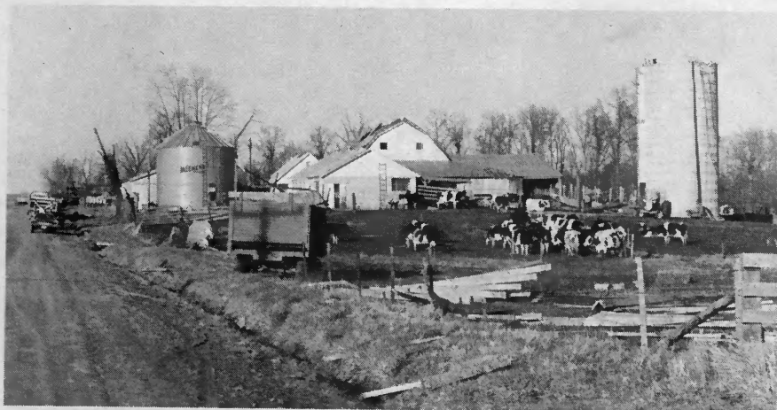
Youngblood's dairy farm, south of Orchardville, suffered severe damage. Most buildings were either damaged or destroyed.
