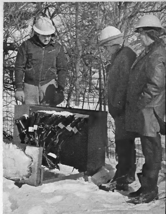
Inspecting an underground junction box where a circuit from the substation switches from underground to overhead distribution are, from left, Richard Kincaid, line foreman; Morris Deul, manager, and Simon Vandersnick, president of Farmers Mutual Electric Company.
