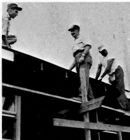
Another electrically heated home is being added to the growing list served by Rural Electric Convenience Cooperative Co. This is the new home of Harry McGinnis, Jr., of rural Raymond. Contractor Robert Johnson (left) of Raymond is directing construction of the 2,000-square-foot home with assistance from Harry McGinnis, Sr. (center) and the proud new homeowner.
