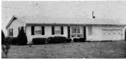
Warren Dempsey Carlyle Ceiling Cable
