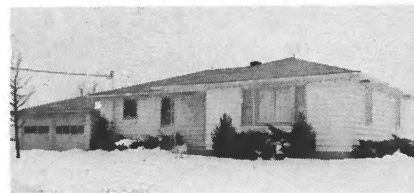
Robert Kellermann Carlyle r.r. 4 Ceiling Cable
