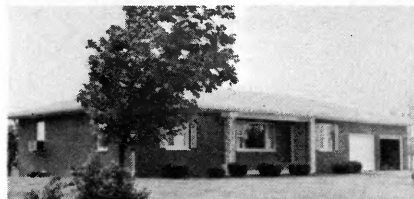
Edward Meier Hoffman Ceiling Cable
