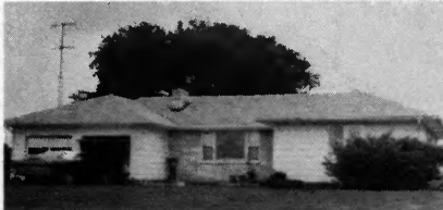
Dennis Emery Centralia Ceiling Cable
