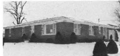
Ray Pingsterhaus Carlyle r.r. 3 Ceiling Cable
