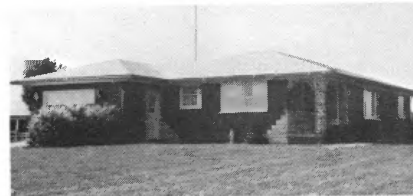
Norbert Jansen Germantown Hot Water Baseboard
