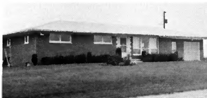
Larry Spanley Trenton Ceiling Cable
