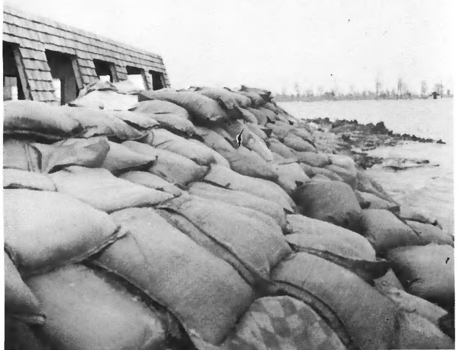
Hundreds of sandbags surround the West Access Marina Restaurant at Lake Carlyle where heavy April rains raised the lake to its highest level.
