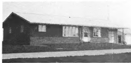
Carl Nottmeyer Centralia Ceiling Cable
