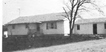
William Nottmeyer Centralia Ceiling Cable
