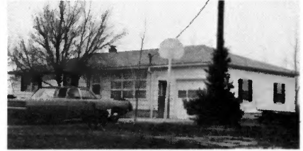
Burnell Warnecke Breese Ceiling Cable
