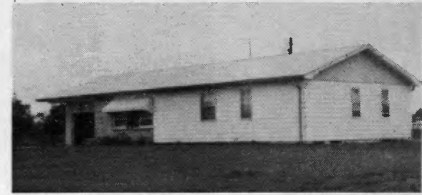
Leroy Mensing Centralia Ceiling Cable
