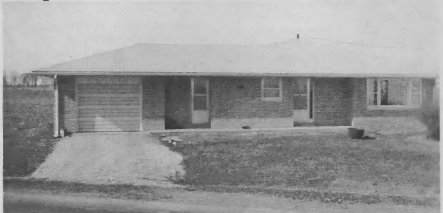
The new all-electric Gold Medallion home of Mrs. Mary Blankenship is 10 miles north of Taylorville.
