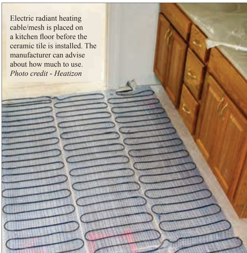
This electric floor radiant heating kit contains heating cable spaced properly in a mesh casing. This is ideal for tile floor applications. Photo credit - Warmly Yours
