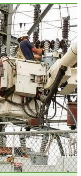
To help with increasing reliability and reducing outages, WIEC periodically does routine maintenance on our equipment. Here, one of our linemen is replacing the breakers at the Carthage substation. Although Prairie Power Inc. owns the substation, the distribution breakers located in the substation belong to WIEC, and we maintain them.
