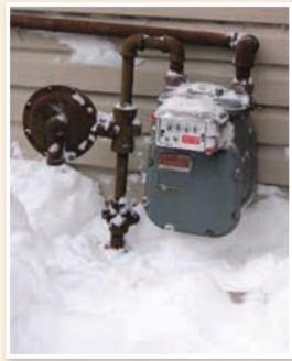
As you're shoveling sidewalks and driveways this winter, remember to check your natural gas meter and pipes for drifted snow, top, which can cause problems. When exposing the meter and pipes, avoid using a snow blower. Instead, aently remove snow and ice from the area. Also remember to clear snow away from furnace intake and exhaust pipes.
