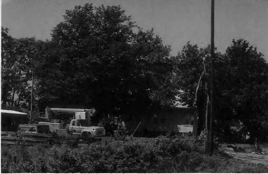
Opposite page: Damage to just one pole can cut electric power to a large area. This page: The bright yellow service trucks of electric cooperatives were common in the affected region.
