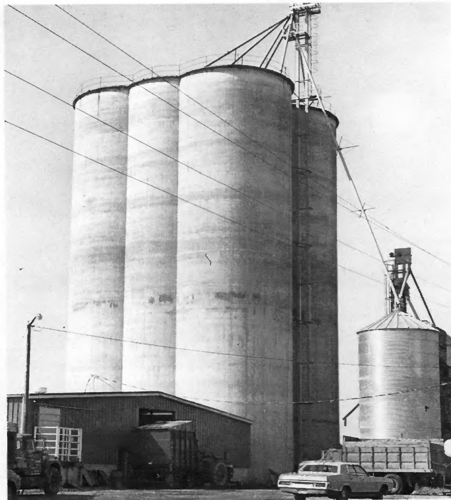
Grain drying, storage and confinement house are all interconnected. As Kissner explains it, everything is done with the push of a button, thanks to electricity.
