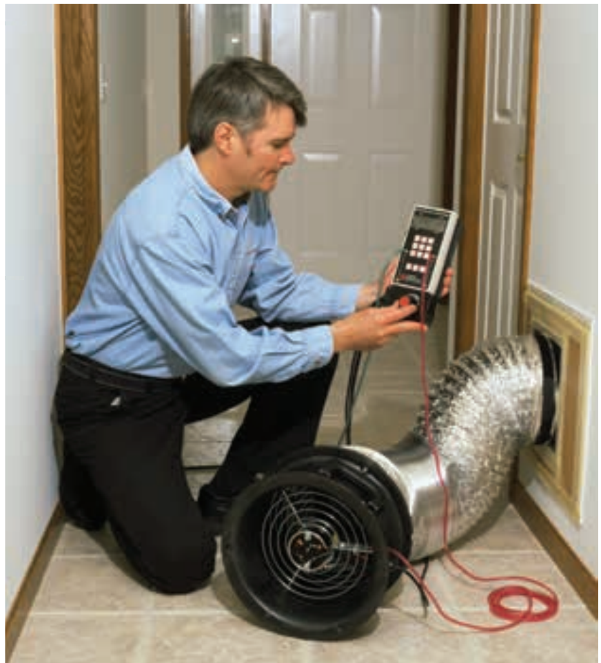
A Duct Blaster test can show you how leaky your ductwork is.
