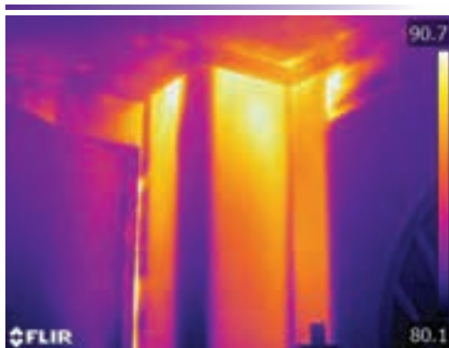
A flue chase for the furnace and water heater in a basement. It is a 2-foot by 2-foot hole from the attic to the basement in a two story home.
