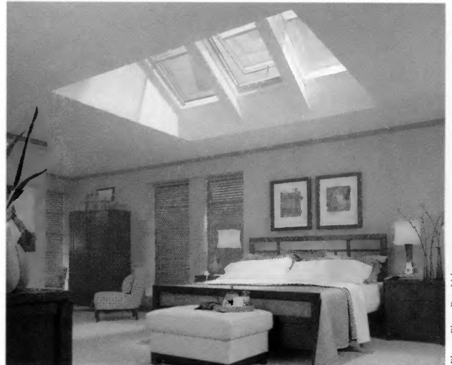
This bedroom uses a combination of one venting and two fixed skylights. Mini-Venetian blinds are installed in the gaps between the multipanes.
