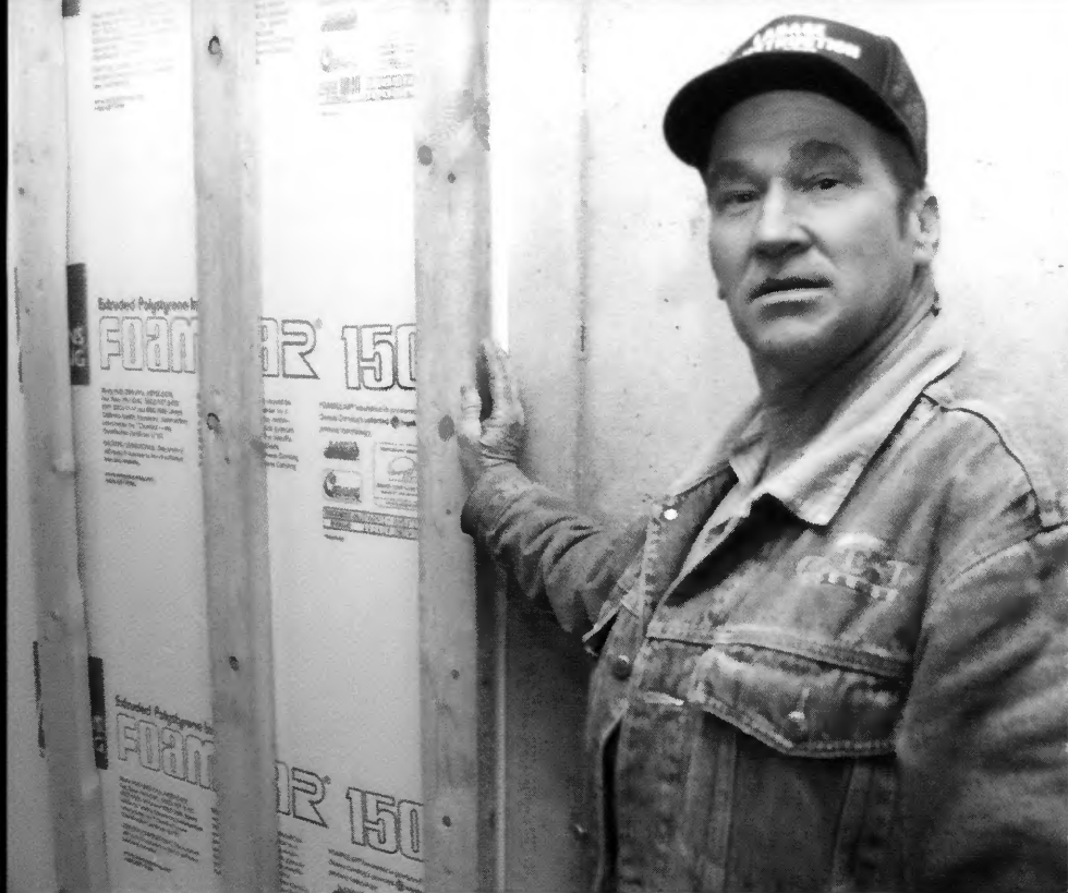
Weldon Ladage, Owner of Ladage Construction, says you only get one chance to seal out air infiltration, and that's before the dry wall is installed.
