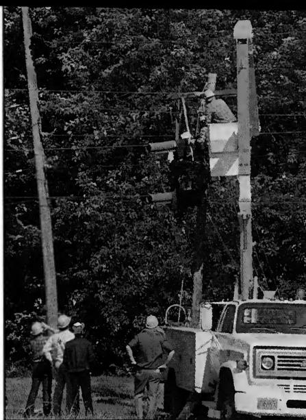
*Opposite page, linemen work on simulated "live" lines during the Hot Line School. Note heavy gloves, "coverup" materials on lines and nonconductive hotsticks hanging within easy reach. At left, linemen on a pole work under the careful supervision of an instructor in a bucket. Below, an instructor shows how to make ties.*
