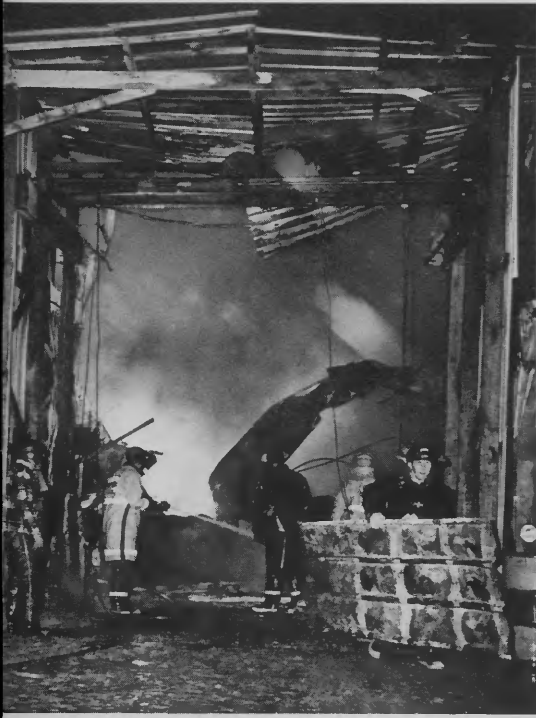
AT LEFT: Firemen hose down the remaining shell of the building.
