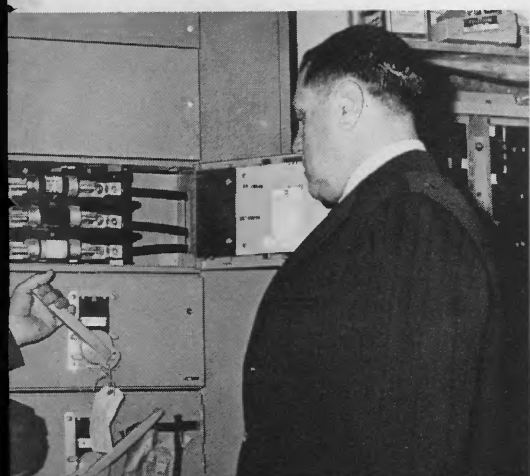
ABOVE: The beautiful sanctuary of the Apostolic Christian Church. The church will be heated and cooled by one system—a heat pump. BELOW LEFT: Joe Crosno, power use adviser for Corn Belt Electric Cooperative, Bloomington, inspects one of the heat pump units on the church's roof. BELOW: Crosno explains the workings of the heat pump's fuse box to Alden Nussbaum, a member of the church's building committee.
