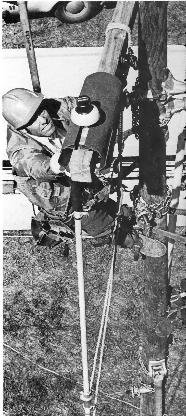
ABOVE: Silhouetted by the midday sun, linemen learn the use of "hot sticks" at the outdoor training laboratory. CENTER: Proper tools and safe methods make working on live, energized electrical lines possible. These two linemen are rigging a pole so they can do repair work on the crossarm.
