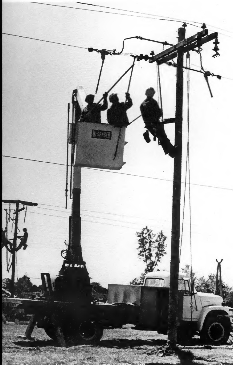
ABOVE: Silhouetted by the midday sun, linemen learn the use of "hot sticks" at the outdoor training laboratory. CENTER: Proper tools and safe methods make working on live, energized electrical lines possible. These two linemen are rigging a pole so they can do repair work on the crossarm.
