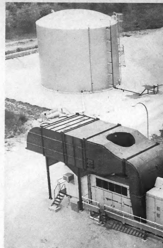
WIPCO, finally was able to line up a supply sufficient to fill the turbine's 300,000 gallon storage tank. This sounds like a lot, and it was fully adequate to test the machine and prove it to be in good working order. But, a 21,000 kilowatt combustion turbine consumes oil in what the average person would consider prodigious quantities. In fact, five days of continuous full load operation would exhaust the storage tank completely.
