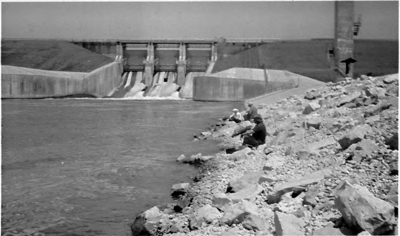
*Shelby Electric Cooperative, Shelbyville, provides power to operate the gates of the Shelbyville dam. The dam's minimum flow is 50 cubic feet of water per second with as much as 1,200 cubic feet per second following a heavy rainfall.*
