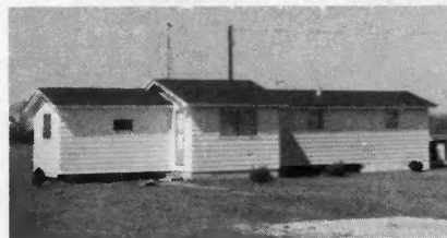
Mr. and Mrs. James Boldrey 3½ Miles Southwest of Mt. Vernon 706 Sq. Ft. of Living Area Rebuilt Storm Damaged Mobile Home 1970 Contractor—Art Puckett Electrical Contractor—Art Puckett
