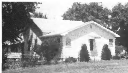
Mr. and Mrs. Frank Waier 3 Miles West of Ashley New Addition Heated Electrically 1966 484 Sq. Ft. of Living Area
