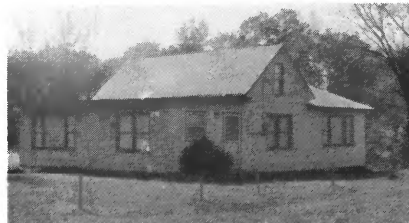
Mr. and Mrs. Edwin Pedtke Radom 1,191 Sq. Ft. of Living Area Converted to Electric Heat in 1971 Electrical Contractor—J. D. Electric
