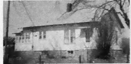
Mr. and Mrs. Luther Hester 4½ Miles South of Mt. Vernon 808 Sq. Ft. of Living Area Converted to Electric Heat in 1962 Electrical Contractor—George Donoho
