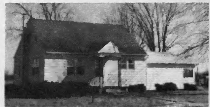
Mr. and Mrs. Richard Phillips 6 Miles East of Centralia 810 Sq. Ft. of Living Area Converted to Electric Heat in 1964 New Addition Heated Electrically 1966
