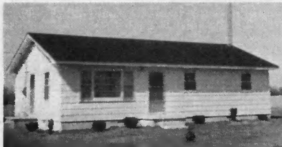
Mr. and Mrs. Marvin Kisner 4 Miles Southwest of Mt. Vernon 1,071 Sq. Ft. of Living Area Built in 1967 Electrical Contractor—Homeowner Contractor—Scott and Shannon
