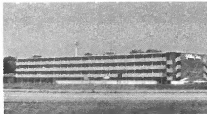
Holiday Inn West Edge of Mt. Vernon Built in 1971 Electrical Contractor—D. C. Electric
