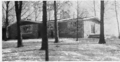
Mr. and Mrs. Carroll Gregory 2 Miles Northwest of Bluford New Addition Heated Electrically 1969 360 Sq. Ft. of Living Area Contractor—Homeowner Electrical Contractor—Homeowner
