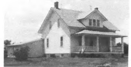
Mr. and Mrs. Robert Heckert 1/2 Mile South of Stone Church Converted to Electric Heat in 1971 1,719 Sq. Ft. of Living Area Electrical Contractor—Weeke
