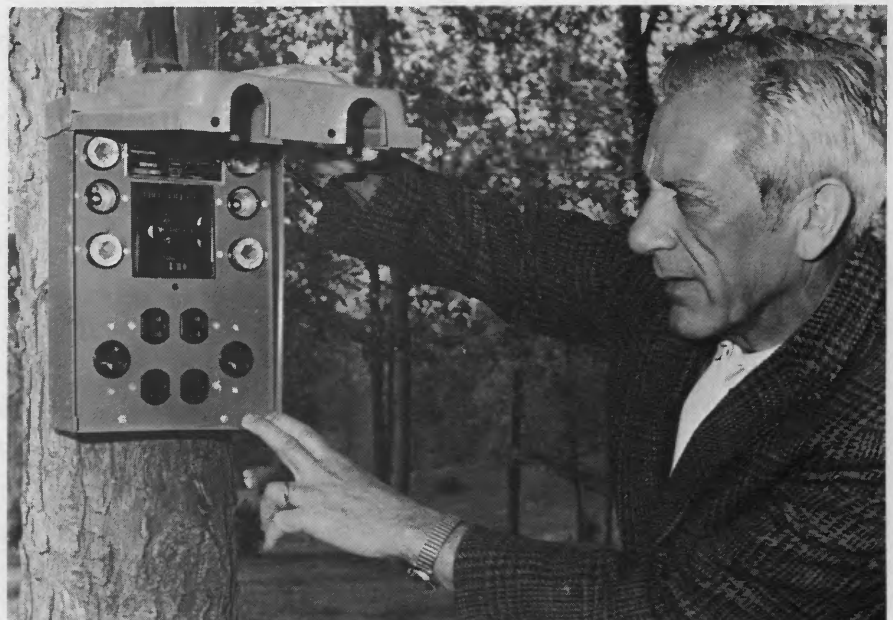
Joe Crosno, power use advisor for Corn Belt Electric Cooperative, with an electrical hook-up for individual campsites.
