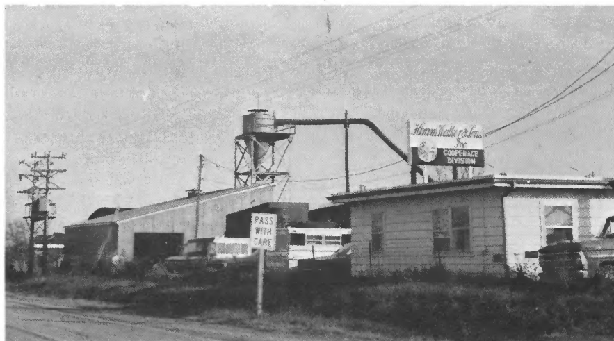
WIEC provides three-phase electric service to Hiram Walker and Sons, Inc. plant south of Hamilton on Highway 96.
