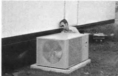
Ron Lowderman prepares a mobile home and connects a three-ton central air conditioner unit.
