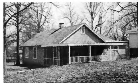
W. A. Pyle, near Carmi 9,600 watts, 2-ton heat pump
