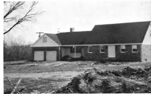
Norman Fechtig 2100 sq. ft., ceiling cable 16,800 watts est. op. cost, $198.10
