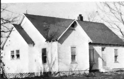
James E. Fenton, Wayne City 816 sq. ft., baseboard 8,000 watts est. op. cost, $107.82
