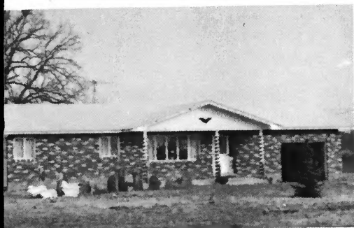
Glen Miller, Wayne City 1,269 sq. ft., ceiling cable 11,200 watts est. op. cost, $155.02
