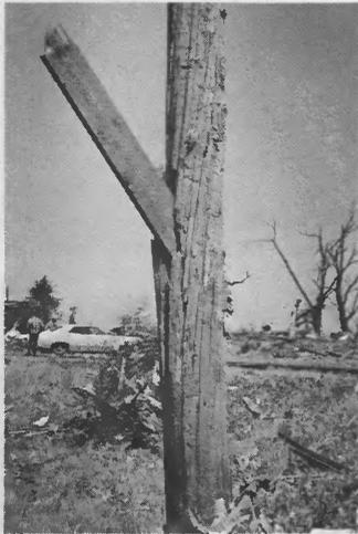
The storm's fury is apparent from this broken board which penetrates an electric line pole.
