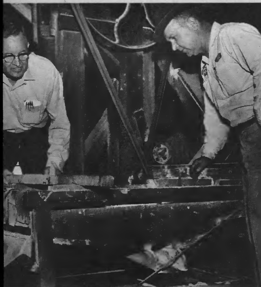
Henry J. Wallace (left) and William D. Musgrave examine part of the mill machinery.
