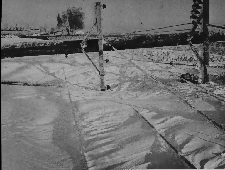
Transmission line falls prey to storm.
